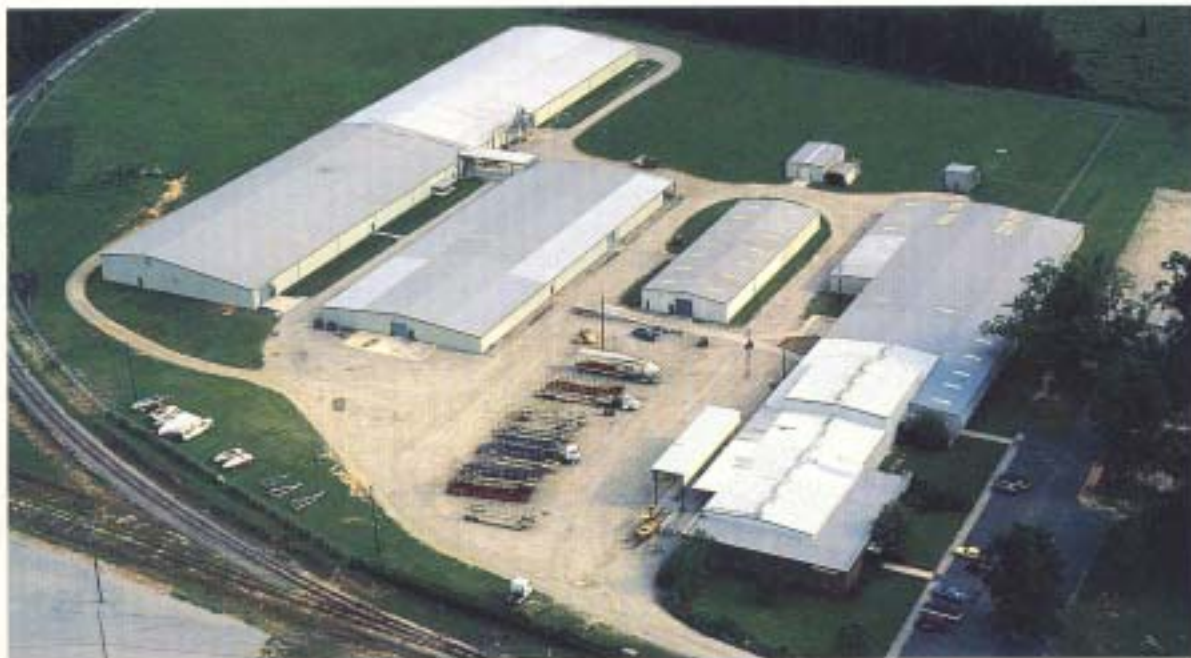
With over 200,000 square feet of production and research and development facilities, Stingray continues to expand into the 21st Century.
